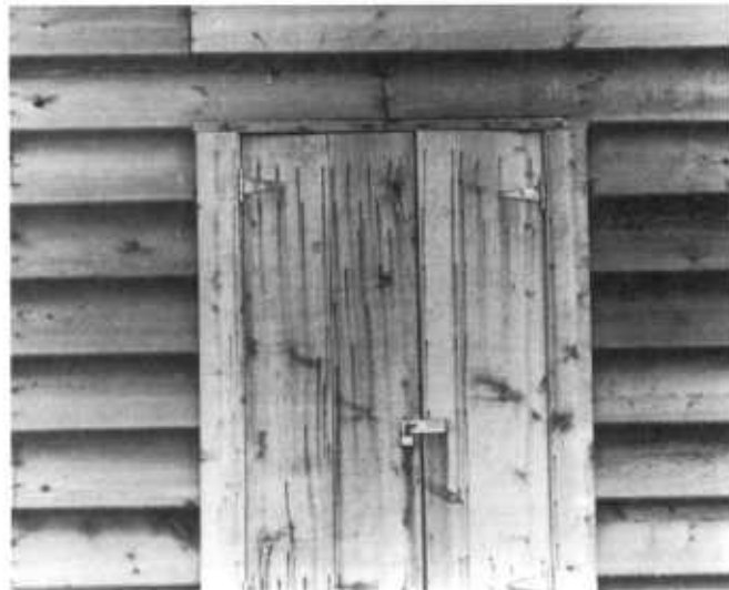
Figure 39 —Blue-black discoloration resulting from the use of ferrous nails.
