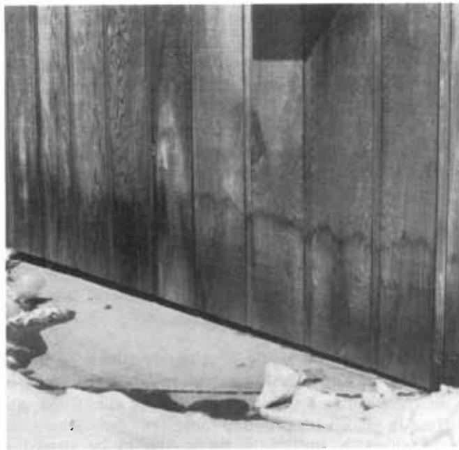
Figure 6 —Rainwater splash on naturally finished plywood siding. Rainwater runs from the roof and wets the siding as it hits the concrete sidewalk.
