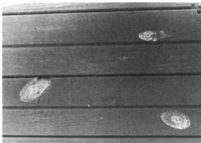
Figure 41 —Exuded pitch from knots and pitch pocket on siding.
