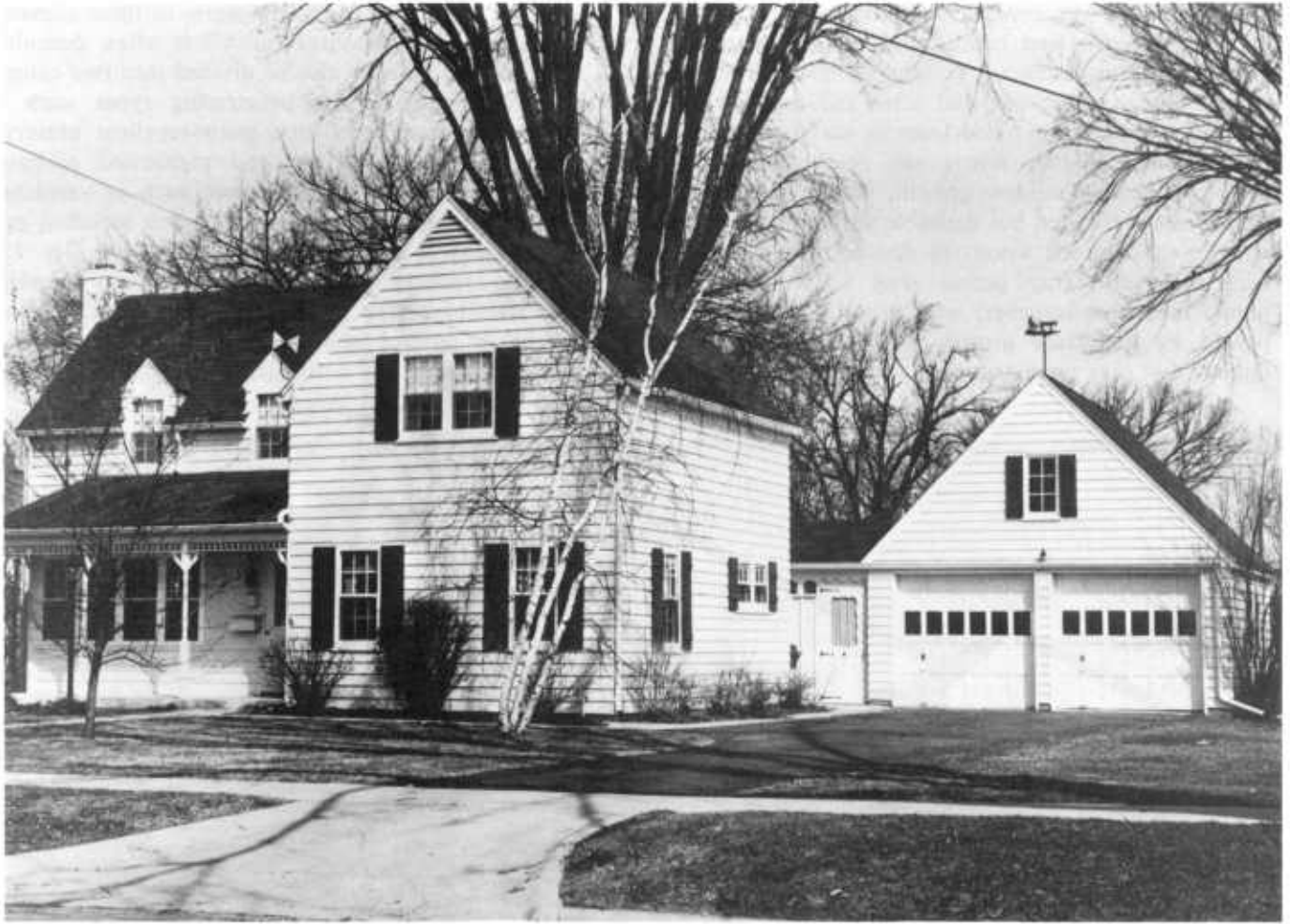
Figure 20 —A 110-year-old house, re-sided in 1930 and maintained with good painting practices.
