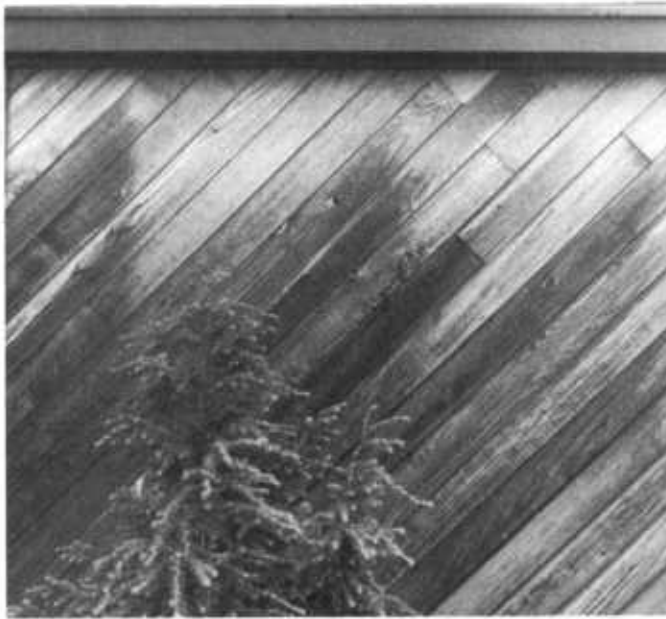
Figure 16 —Mildew on naturally weathered siding.
